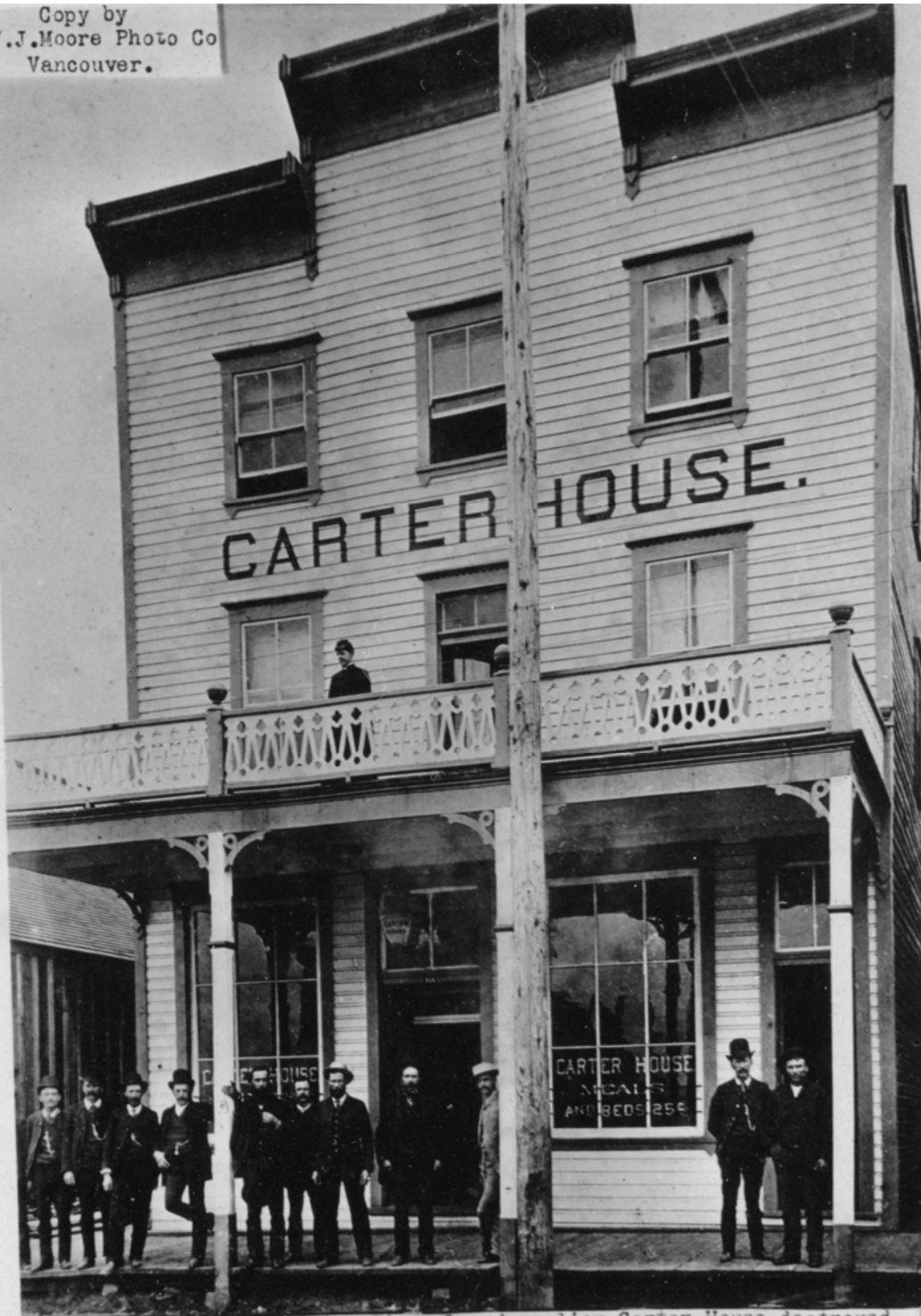
Famous hostelry, 166 Water St, replaced earlier Carter House destroyed in great fire 1886 two weeks after opening, first three story building in Vanc'r. Demolished 1921-2. quartered police enforcing suspension city charter, Chinese Riots 1887. On verandah, Mrs (Margaret J) Carter, 3rd from left: C.E. Taggart, 4th Chas E Doering, 5th Lewis Carter, owner, 7th John L. Carter, brother. Copyright W.F. Findlay, 244 E 11th St.
